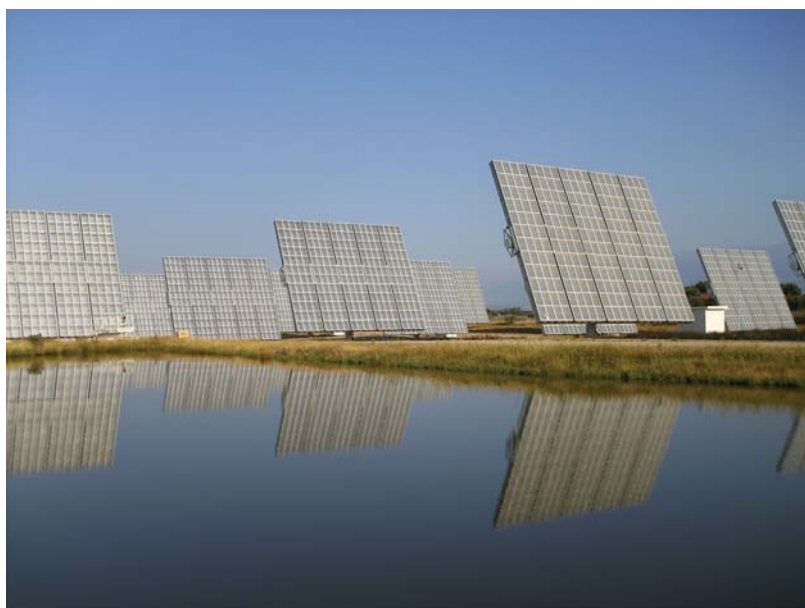
Plate 2 Figure 10.2 Evolution and commercialization of the Fresnel lens technology initiated in Sandia Labs (1976): 750 \text{kW}_p plant, manufactured and installed by Guascor Fotón in Cáceres, Spain, 2007) (Courtesy Guascor Fotón)
