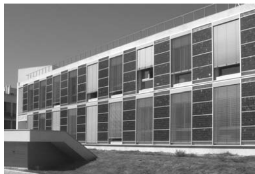
Figure 23.9 Façade integrated PV at the University of Technology in Lisbon (Portugal). Reproduced with permission by H.F. Kaan
