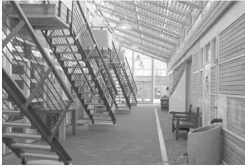
Figure 23.19 Corridor in the Centre for Sustainability De Kleine Aarde in Bostel (The Netherlands). The space is unheated and naturally ventilated. The 6.7\text{ kW}_p PV system with transparent modules has a double function and reduces the heat load by around 70%. Reproduced from Reijenga T, Böttger W, Proc. 2nd World Conference on Photovoltaic Solar Energy Conversion , pp 2748–2751 (1998) with permission by NOVEM, R Schropp [10]
