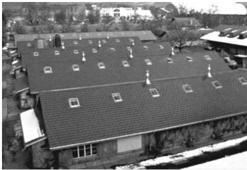
Figure 23.20 The 80.5\text{ kW}_p Atlantis Sunslates on the roof of the historic horse stables in Bern (Switzerland). The color and texture matches so well that this PV system was allowed on a protected historic building. Reproduced with permission by Atlantis Solar Systems Ltd
