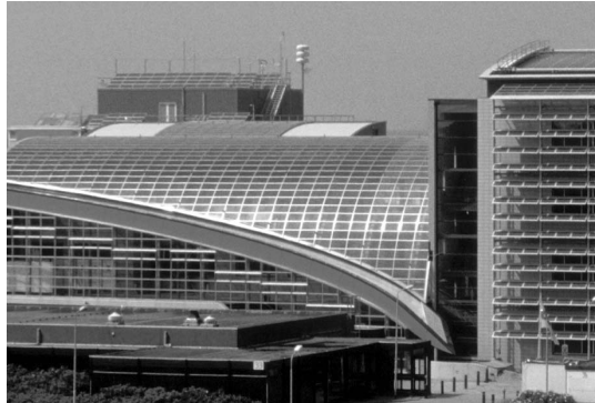
Figure 23.44 This building, at ECN in Petten, The Netherlands has a 43 \text{ kW}_p PV system integrated into the conservatory roof. The conservatory acts as a parasol in front of the offices, thus eliminating the need for air-conditioning in a moderate climate. The building on the right side has a PV shading system (see caption to Figure 23.16). Reproduced with permission by BEAR Architecten T. Reijenga. See Plate 8 for the colour figure
