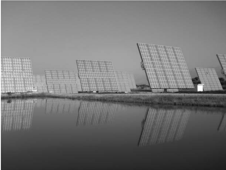
Figure 10.2 Evolution and commercialisation of the Fresnel lens technology initiated in Sandia Labs (1976): 750 kW p plant, manufactured and installed by Guascor Fotón in Cáceres, Spain, 2007) (Courtesy Guascor Fotón) See Plate 2 for the colour figure
