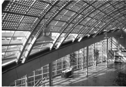
Figure 23.8 Interior view of the conservatory with integrated 43 kW p transparent BP solar modules in ECN Building 42 in Petten (The Netherlands). Reproduced with permission by BEAR Architecten T. Reijenga. See Plate 8 for the colour figure
