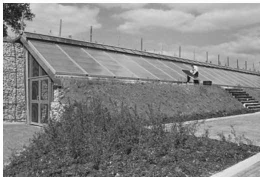
Figure 23.7 PVT modules in the demonstration project at RES UK in Kings Langley, Great Britain. Reproduced with permission by H. F. Kaan
