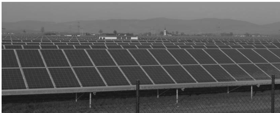
Figure 19.12 Currently one of the world's largest utility scale system (fixed mounting), 54 MW p incorporating 225 000 Si modules and covering 1.3 km 2 , in Strasskirchen, Germany (Courtesy of Raymond Hudson, BEW Engineering)
