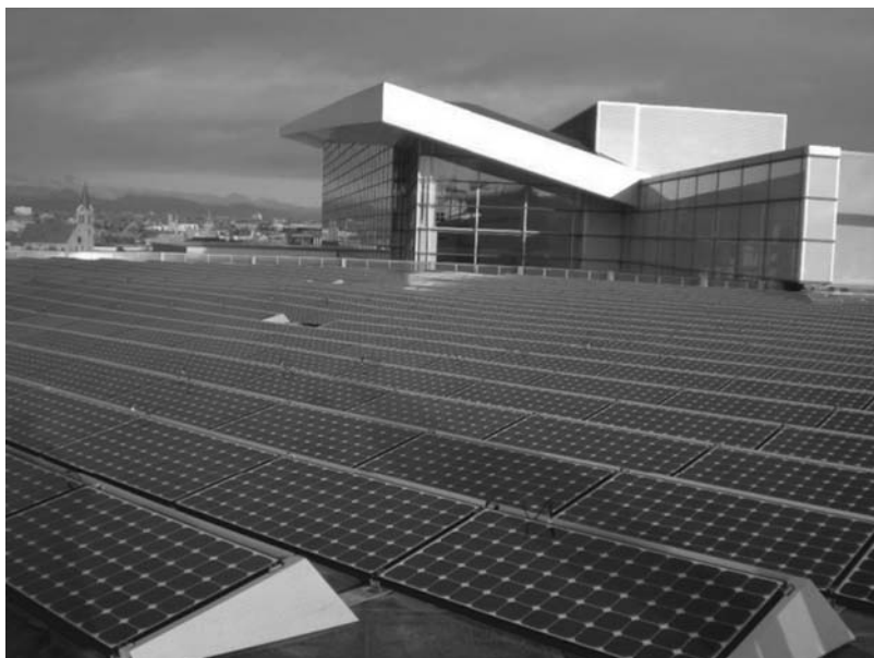
Figure 19.11 Denver, Colorado 300 kW p commercial grid-tied rooftop ballasted system (Courtesy of Brad Eccles, BEW Engineering)
